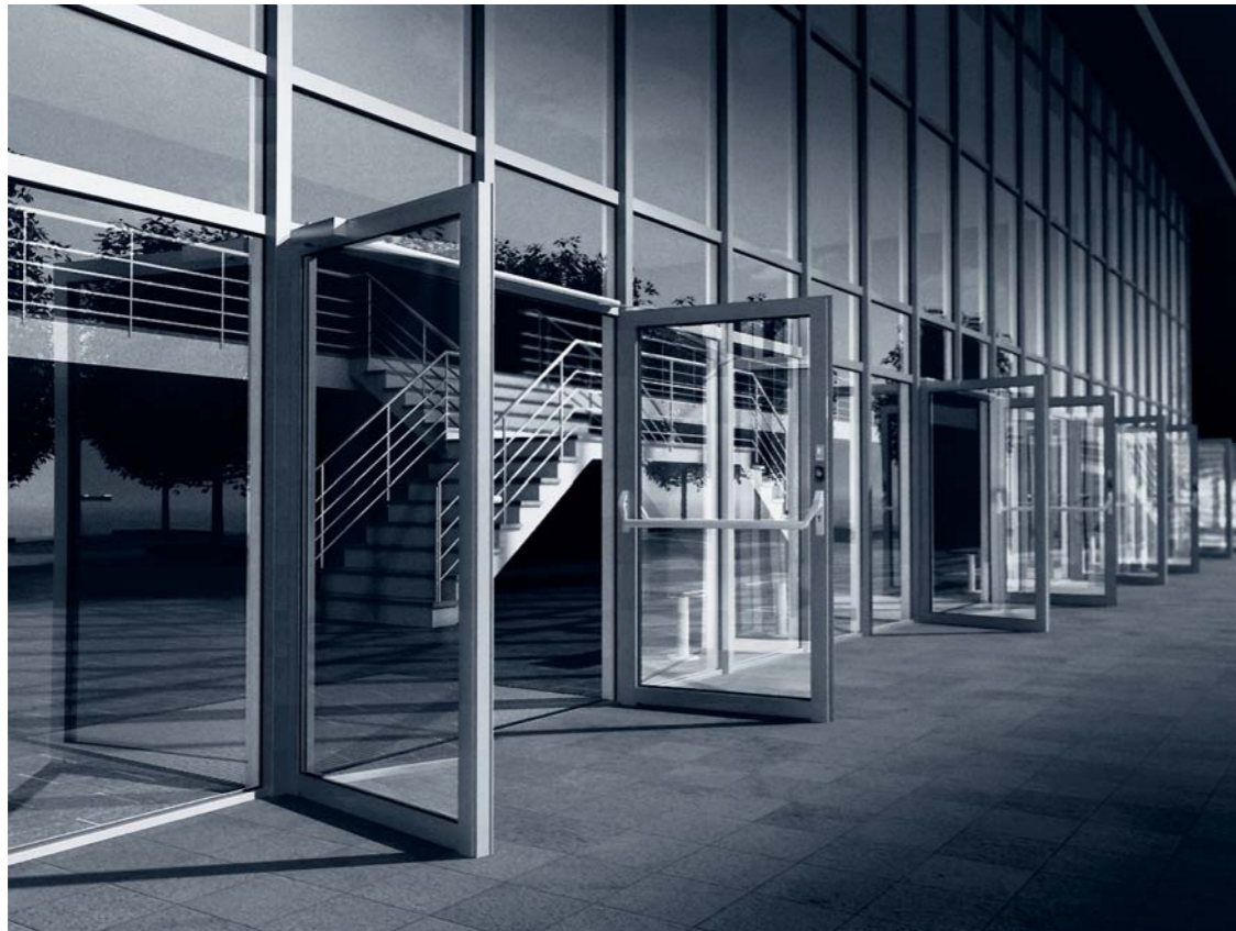
Fachada cortafuegos con salidas de emergencia integradas Fire-resistant façade with integrated emergency exit doors
